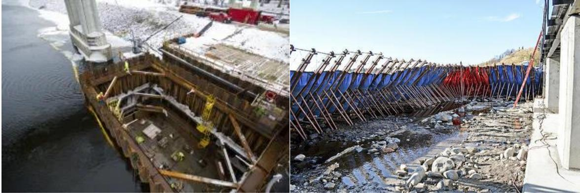
*Figure 2: Braced and Portadam Cofferdam*
