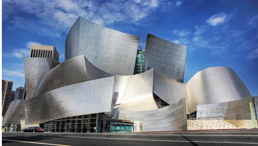
Figure 6: Using steel allows the Walt Disney Concert Hall to achieve this beautiful design
