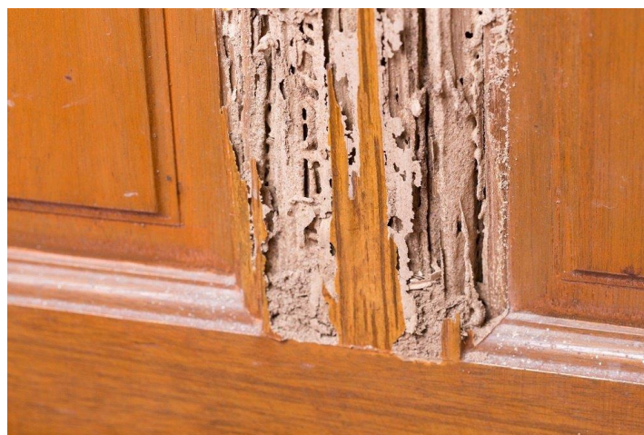
Figure 5: The damage powderpost beetle larvae can do to wood
