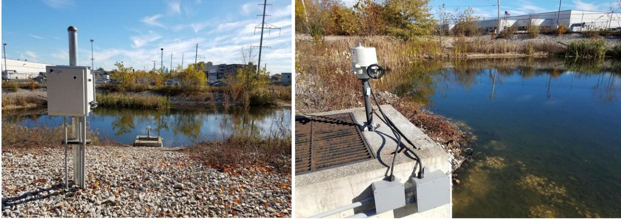
Figures 4a (left) and 4b (right): PWD Retention Pond Real-Time Control System & Valve
