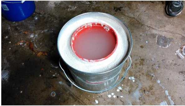
Figure B1. The forge after the mix has been poured into the 6 gallon steel can and the 5 quart plastic bucket has been put in place and filled with water to create the main cavity in the forge.
