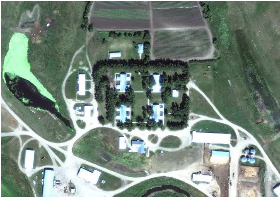
Sandhills Colony in 2011. Four “Brant style” buildings with extensions (no outhouses). Image: Google Earth, 2011, DigitalGlobe.
